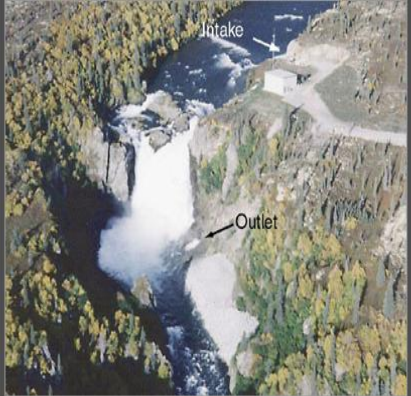
The Tazimina project in Alaska is an example of a diversion hydropower plant. No dam was required.
